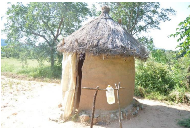
Picture 8: Household toilet constructed using local resources
